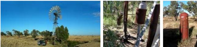
The windmill moves a piston up and down to suck water and then presses it into the poly-pipe.
