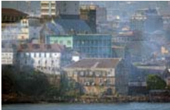
At an old house that looks very run down air-conditioned systems are installed and it seems to be inhabited ....
